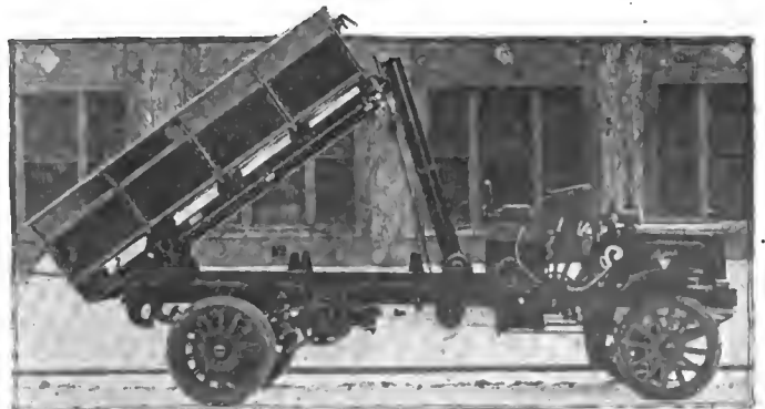
New Packard dumping body, showing same in tilted position
